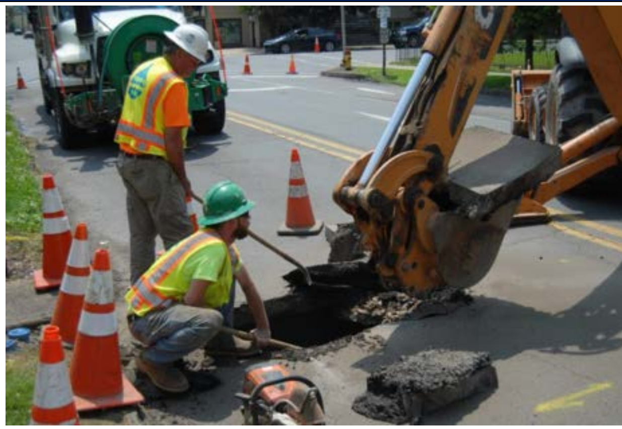
Figure 4.3.8-2 Large Sinkhole caused by sewer break in the City of Williamsport (Danneker, June 1, 2019).
